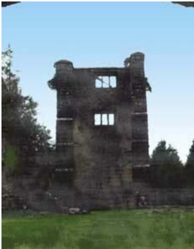
Old Castle Archdale. Photograph courtesy of Fermanagh District Council.
